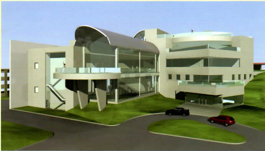
Visual simulation can be used on all projects regardless of size or budget
